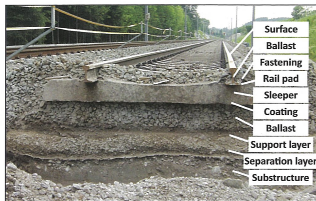
Fig. 1: Example of a modern, multi-layered ballast bed
