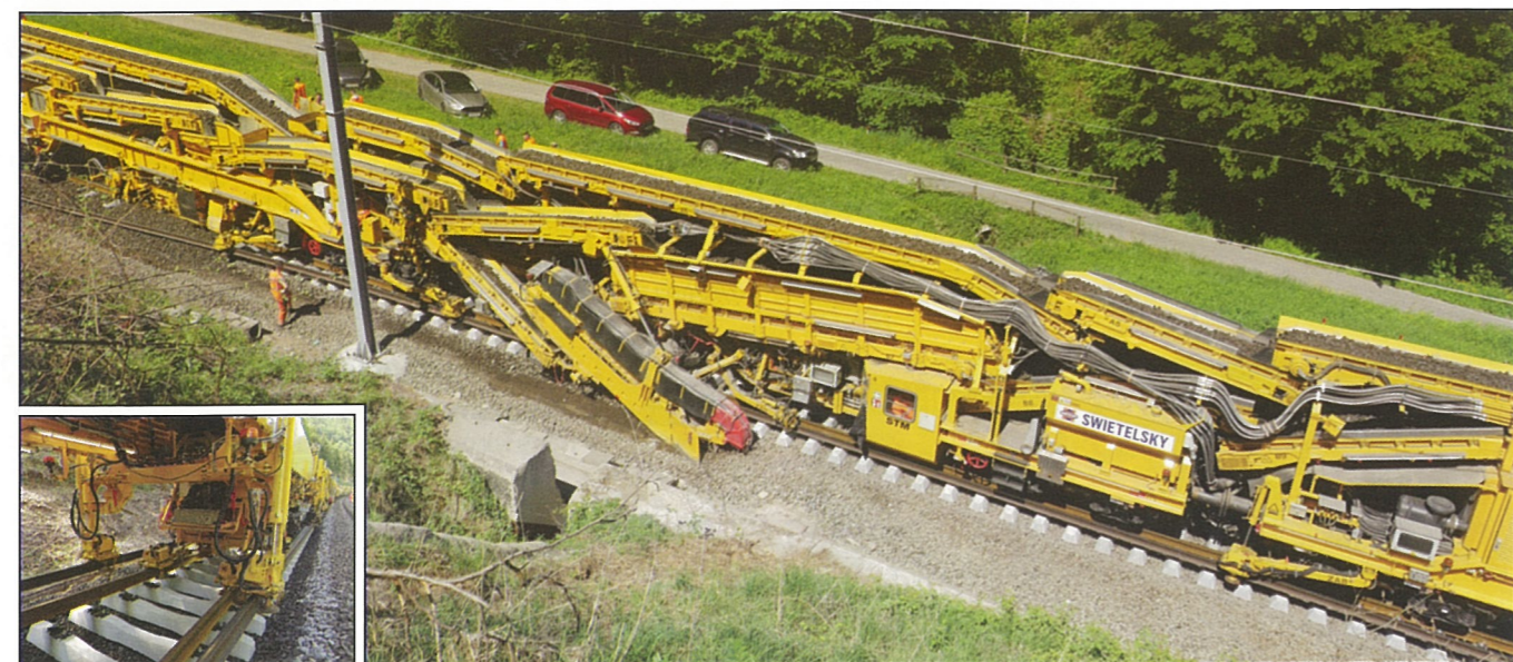
Fig. 8: The RU 1000 S combined track renewal & ballast cleaning machine
