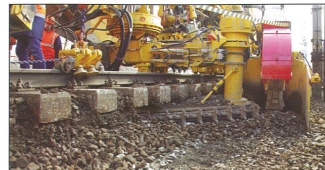
Fig. 9: Non-stop through turnouts (URM 700-2) – no track panel dismantling or access hole digging required
