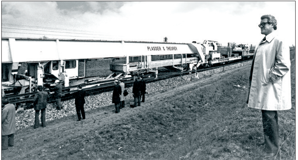
Above: Plasser & Theurer's co-founder Dr Josef Theurer is pictured in 1975 observing a track renewal train in operation. Photograph: Plasser & Theurer.
